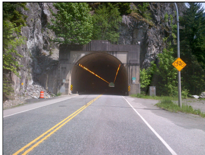
Yale - First of 7 tunnels in the Fraser Canyon
