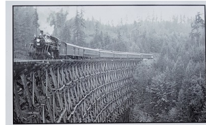
Working Railway Trestle
