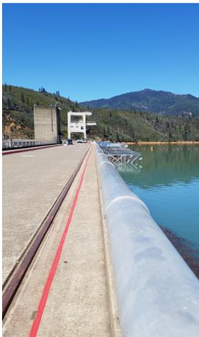
On the left is a picture of the top of the apparatus that was retrofitted a few years ago to allow water to be let in to the turbines from various depths to maintain the "correct" temperature. The "correct" temperature ensures the water leaving the dam is 56°F or less for optimum fish habitat downstream. Pretty clever!
